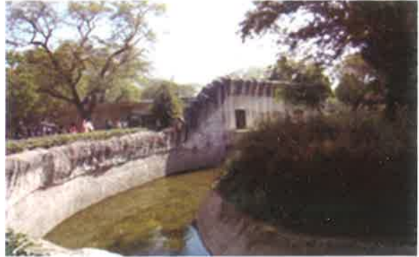
CIVIL STRUCTURES VISIBLE
